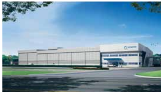
Sumino & Aapico Factory Thailand | 2014
